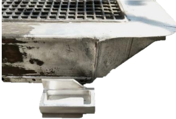
Figure 3: Replacement Flange Before
