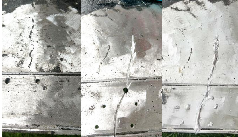
Figure 5: Cracks Are Cleaned, Ground, Repaired and Ground Again
