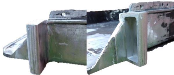
Figure 4: Replacement Flange After
